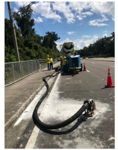
The installation crew at Foundation Professionals of Florida installed 760 cubic yards of AERLITE-iX LDCC to fill the void. They pumped the LDCC through four-inch holes in the roadway surface. Due to its extreme flexibility, the use of LDCC significantly reduced the number of injection points required on the roadway surface.
